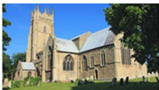
St Andrew's Church Restoration Appeal
